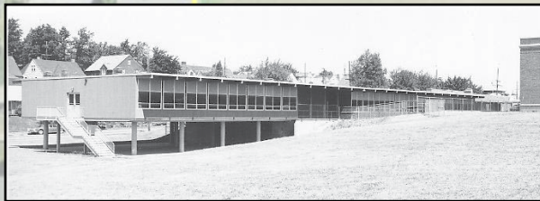
1950s photograph of the 1953 addition to the Hosford School.
