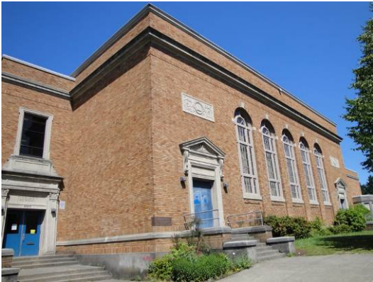
East elevation front entry
