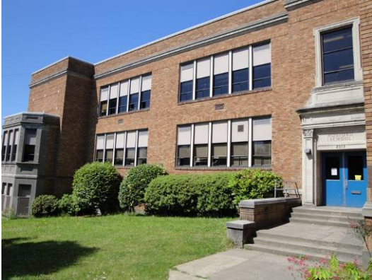
East elevation front entry
